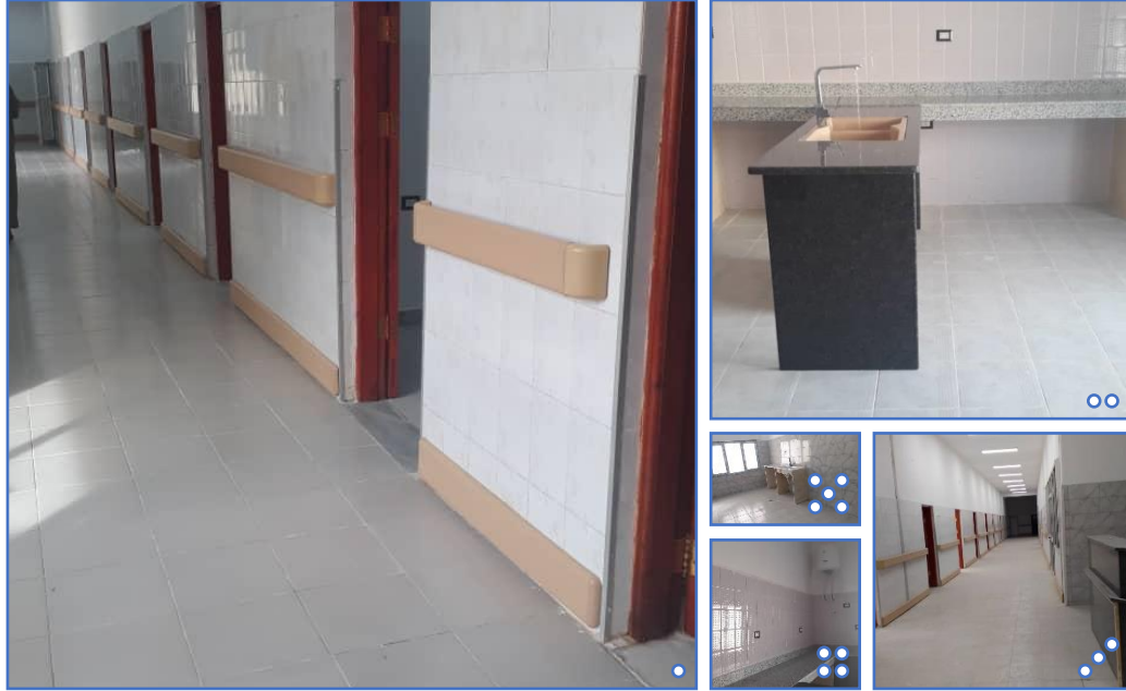
The Alberkat Clinic Centre after rehabilitation
