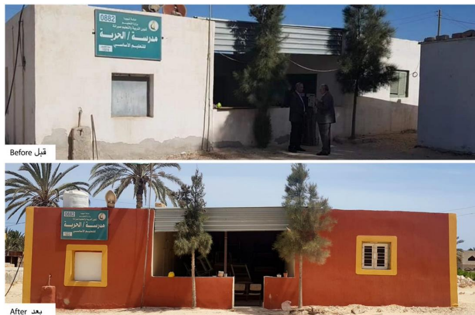
Al-Houria School before and after renovation. ©UNDP Libya
